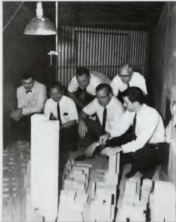
Alan Davenport, Minoru Yamasaki, Malcolm Levy, John Skilling, Jack Cermak, and Leslie Robertson (left to right) crouch inside Cermak's wind tunnel beside a model of Lower Manhattan containing the proposed twin towers, in Fort Collins, Colorado, in 1964. (Colorado State University)
