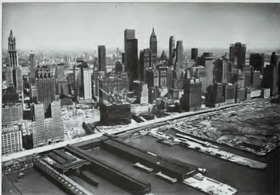
The first section of the Battery Park City landfill, created using soil from the trade center excavation, is seen at right as the north tower begins to rise in May 1969. (Neal Boenzi/ The New York Times )
