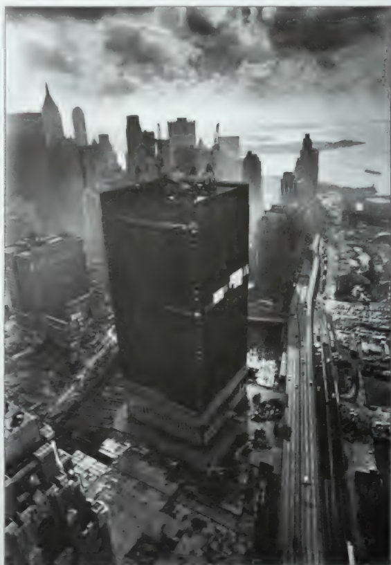
The north tower reaches to approximately the forty-third floor in mid-November 1969. (Edward Hausner/ The New York Times )
