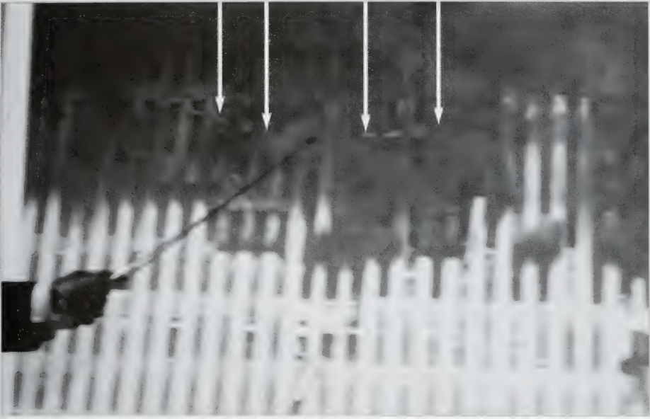
S. Shyam Sunder, an investigator at the National Institute of Standards and Technology, points to a photo showing a sagging floor truss system on the east face of the south tower, twelve minutes before its collapse. (Don Hogan Charles/ The New York Times )
