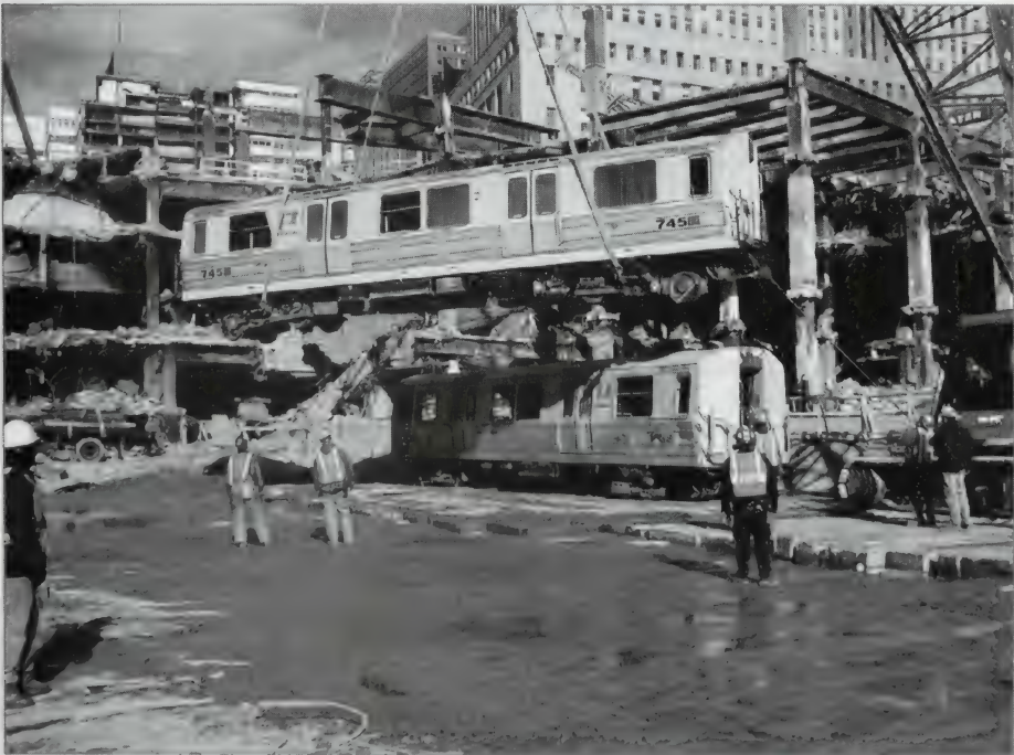
In February 2002, after crews had dug nearly to the bottom of the seventy-foot-deep basement at the World Trade Center, they uncovered PATH commuter rail cars that had been parked at the trade center station at the time of the attack. (Port Authority of New York and New Jersey)
